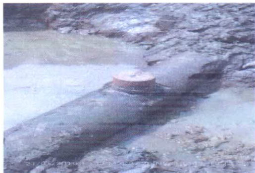
REPAIR WORK DONE BY NAOC REPAIR TEAM
